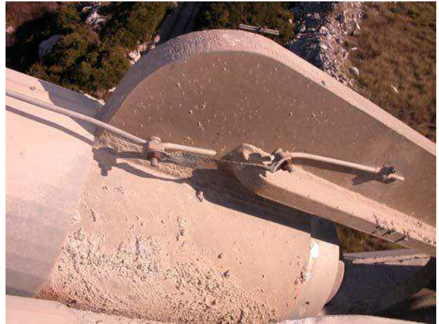
Fig. 5: Flexible lead bonding between the LPS conductor of the stay cable and the support of the stay cable
