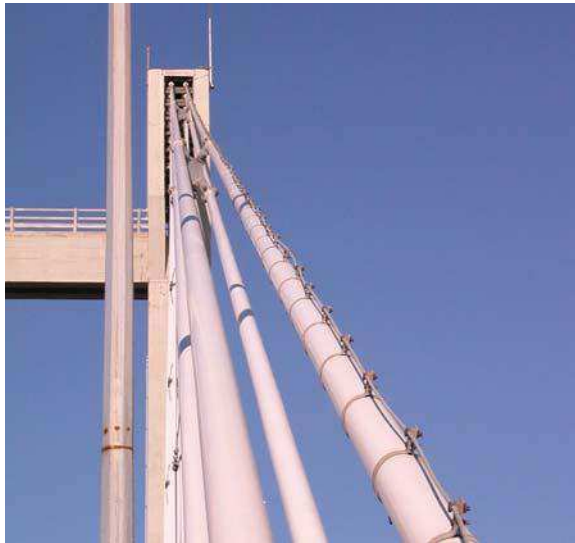
Fig. 3: Protection of the pylons and the stay cables of the Chalkida Bridge
