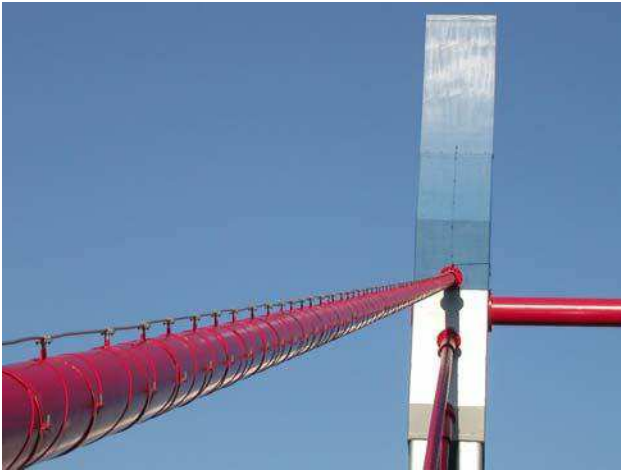
Fig. 7: Protection of the stay cables of the Attiki Odos Bridge
